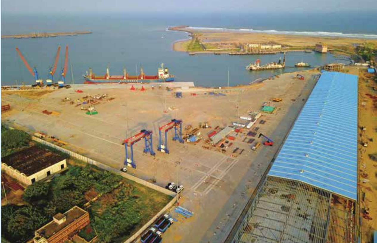
An aerial view of the Paradip International Cargo Terminal
