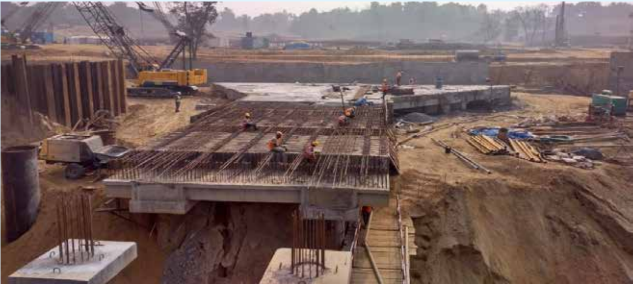
Construction in progress of Multimodal Terminal at Sahibganj
