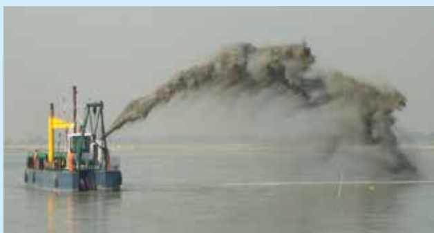
Dredging through Cutter Suction Dredger in NW-1
