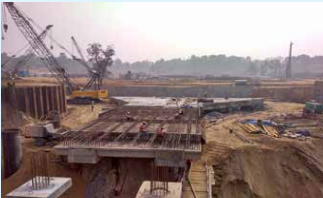
Construction in progress of Multimodal Terminal at Sahibganj
