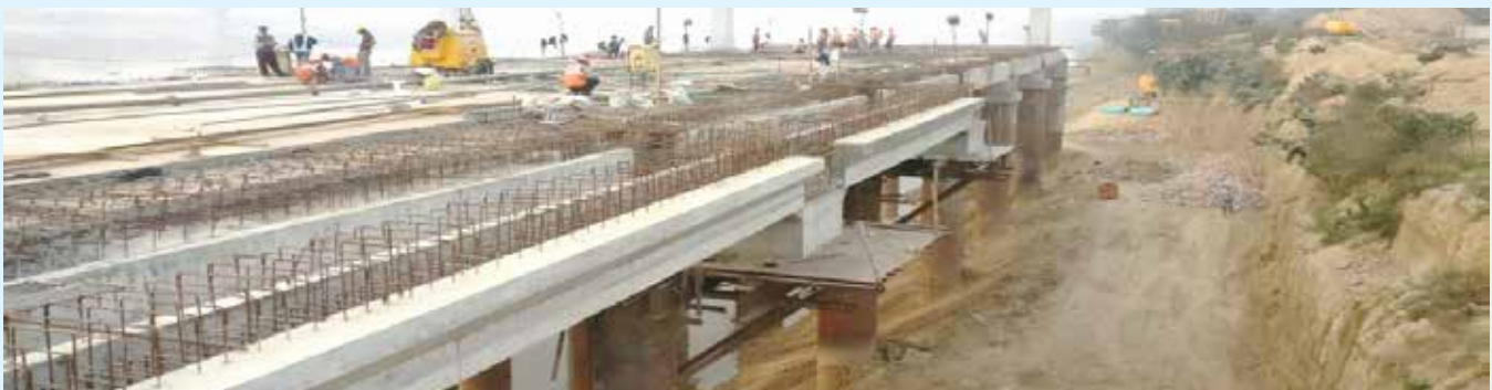
Construction of Multimodal Terminal at Varanasi
