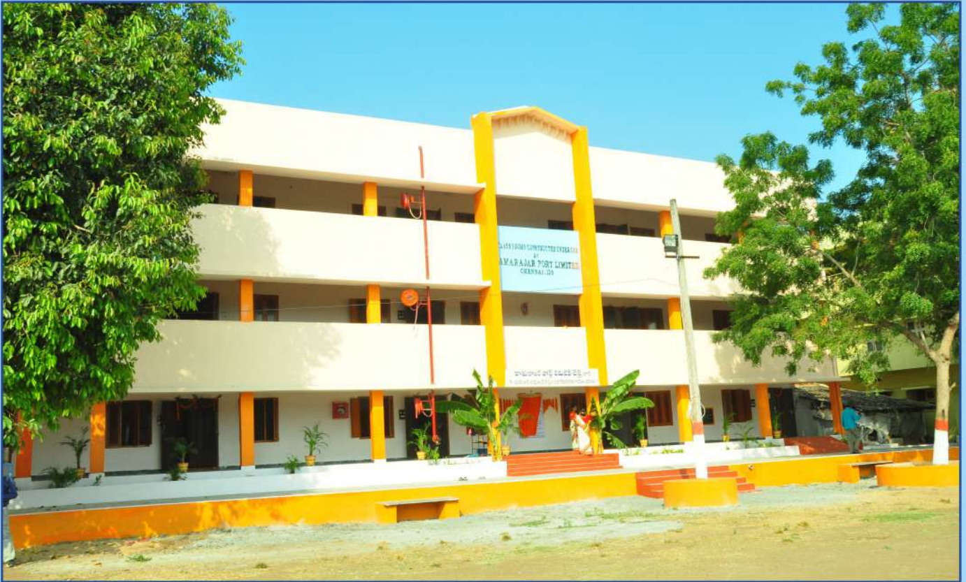
Construction of 12 Class Rooms at Nutakki, Guntur District, Andhra Pradesh under CSR.
