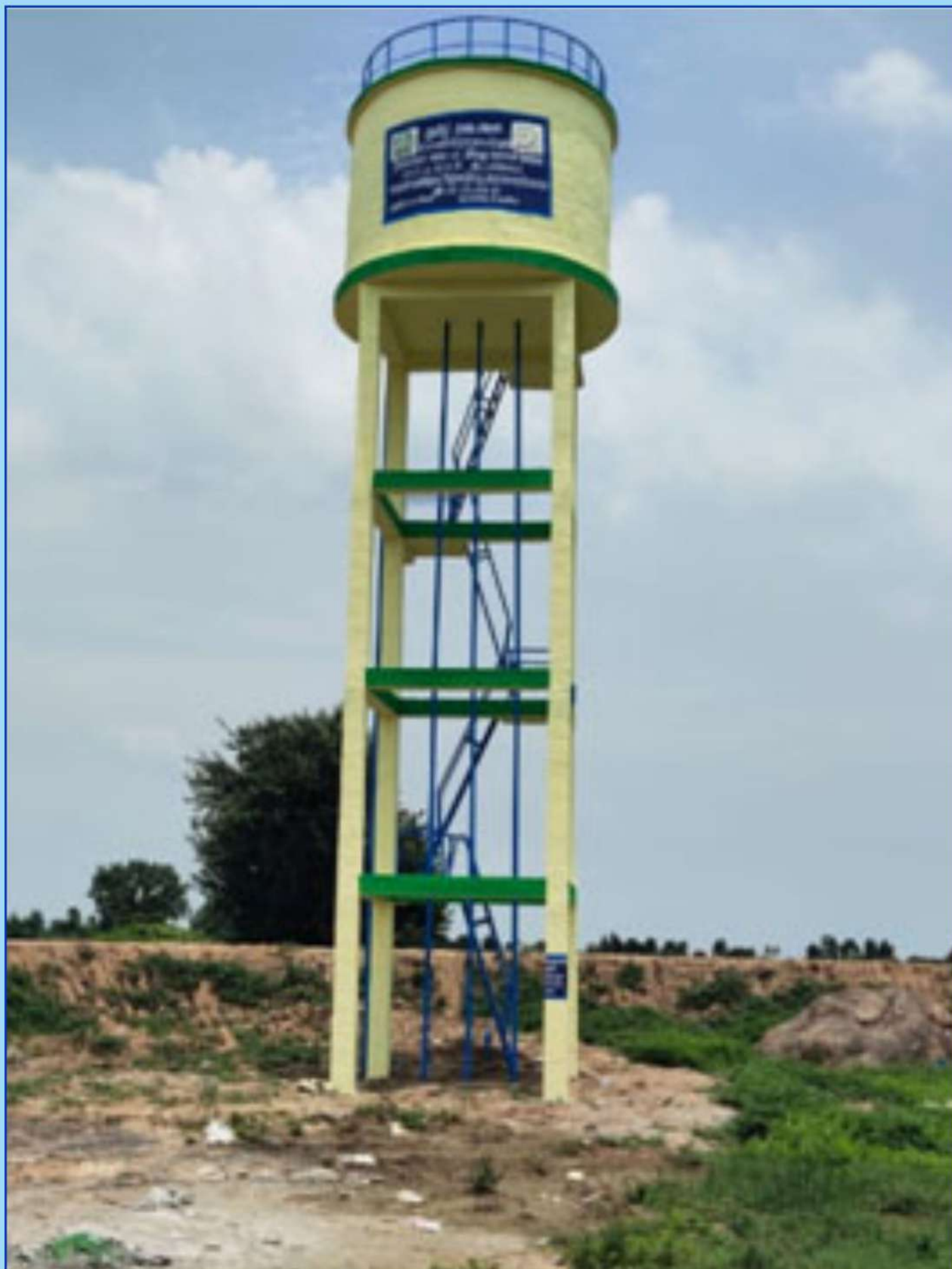
Construction of 30000 Litres OHT in Soambattu east hamlet of Soambattu Panchayat under CSR
