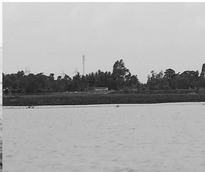
Bank Protection (Phase-I) at Shalukkhali
