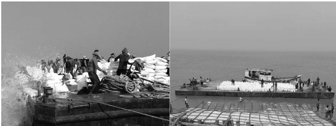
Work of nourishment and re-building of spurs at Nischintapur is in progress
