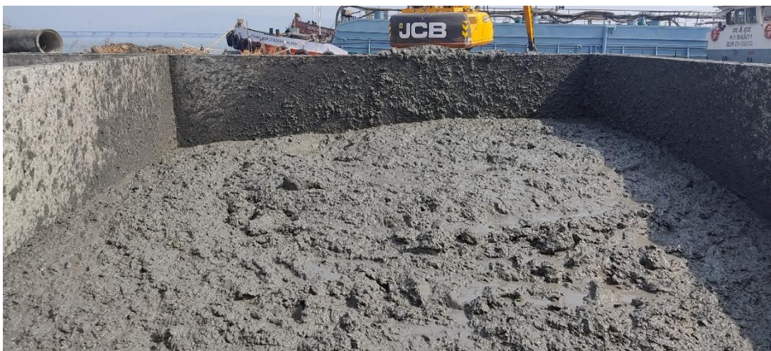
Figure 10. Unloading and Storage of MDS in a Confined Disposal Facility at the site
