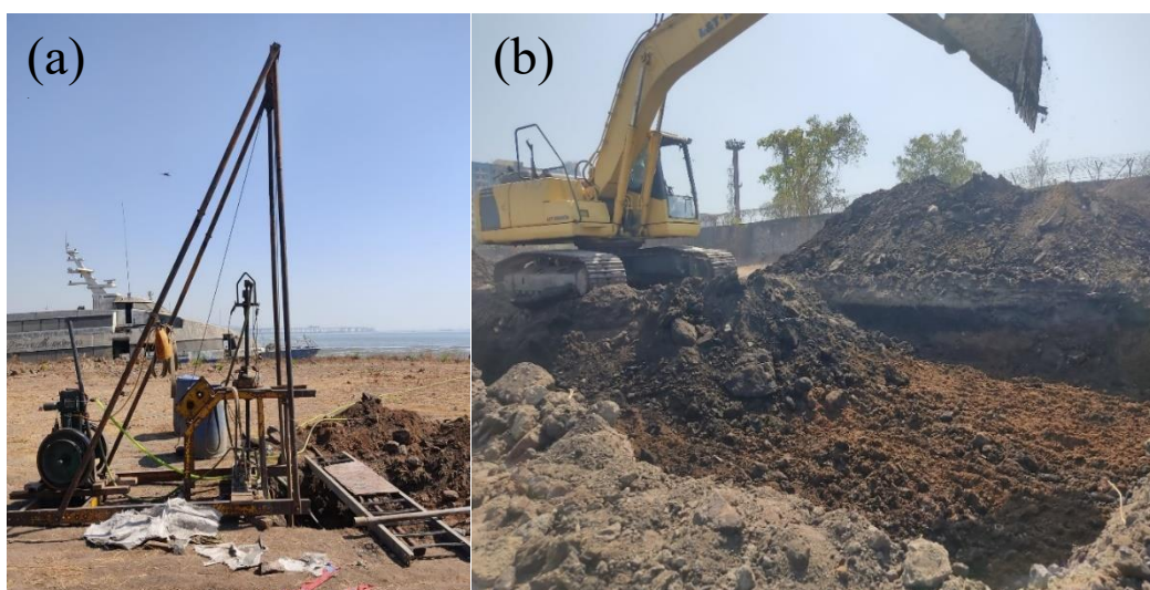
Figure 7. (a) Construction of boreholes at the site (b) Construction of Confined Disposal Facility at the site
