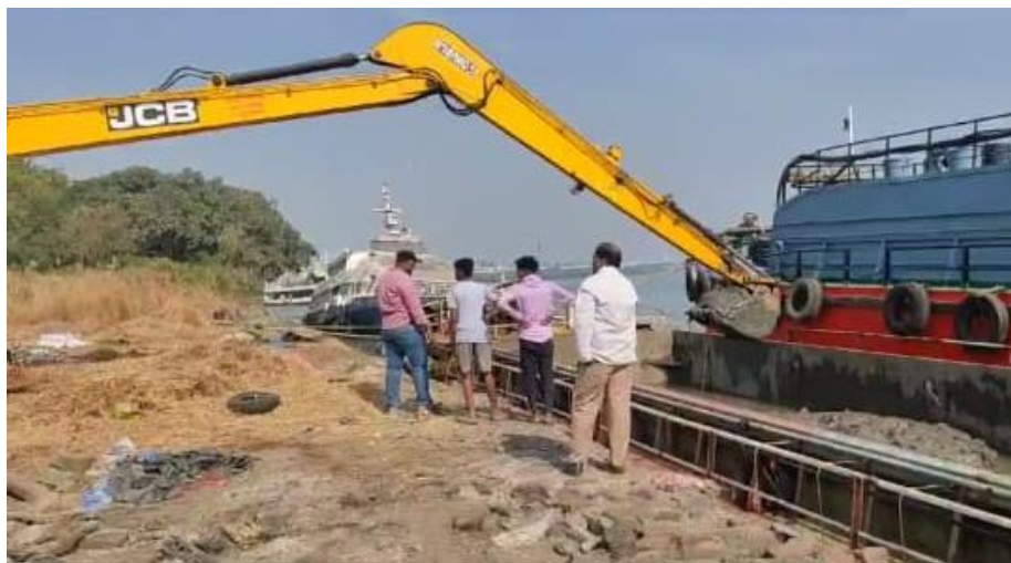
Figure 9. Unloading of the MDS from the barge at the site
