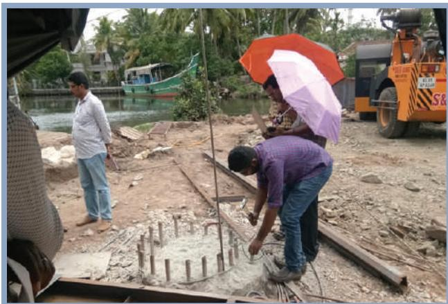
**Piling work by Govt. of Kerala – Construction of lock gate at Thrikkunnappuzha in NW-3**
