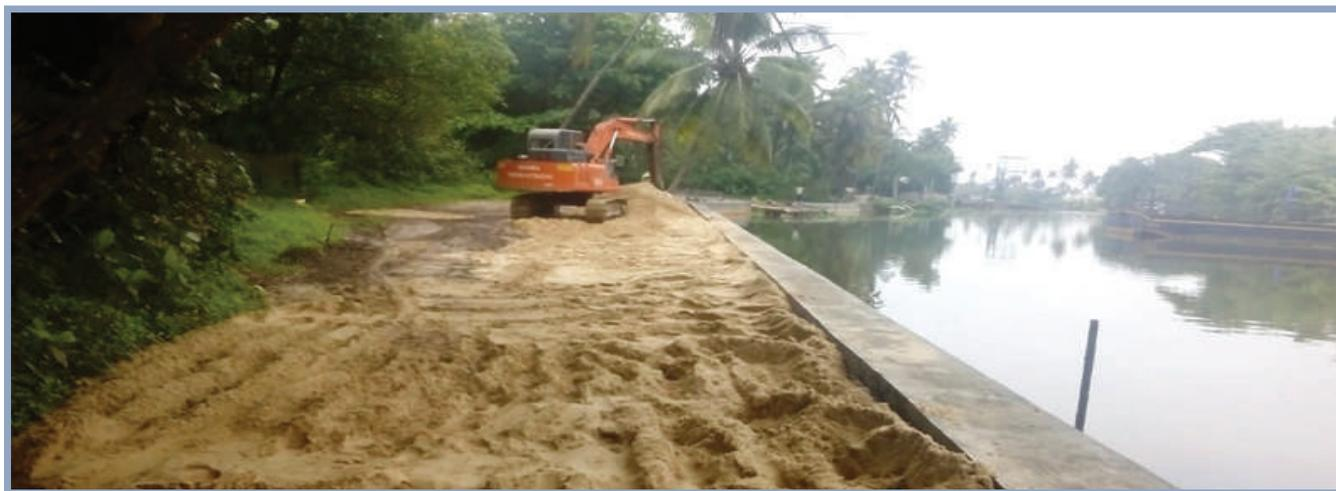
Dredging, widening of narrow canals & bank protection works in Edappallikotta – Kollam stretch of NW-3
