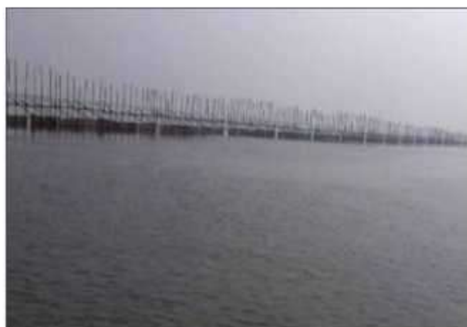
Bandal erected along National Waterway-1
