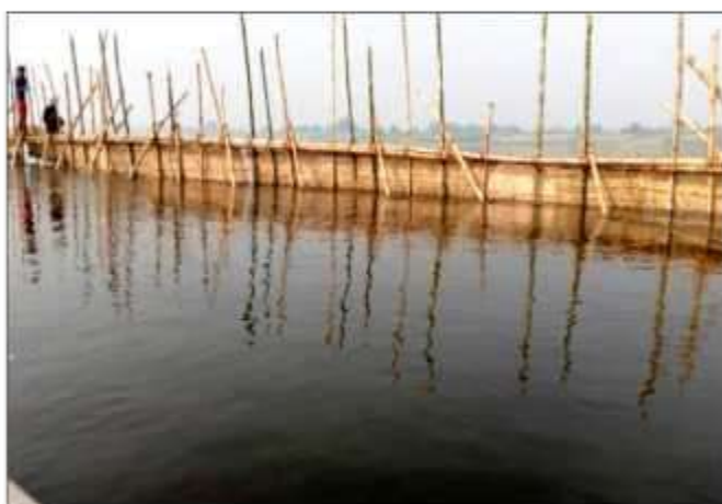
Bandal erected along National Waterway-1
