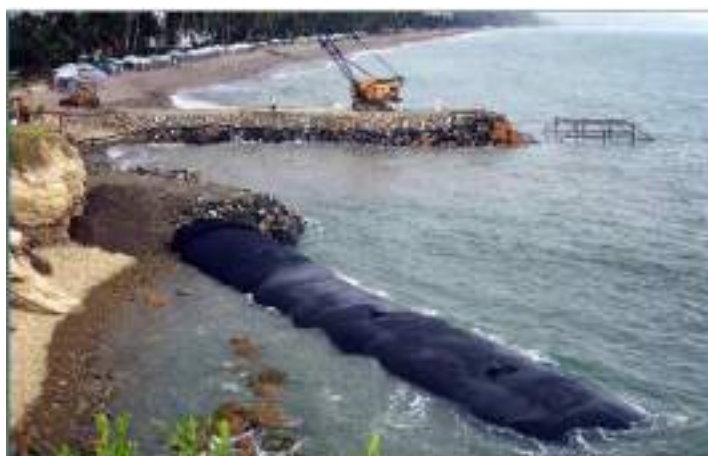
Figure 2.26. Installed groyne using geotube
