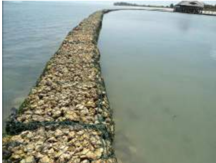
Figure 2.36. Prefilled gabions placed in water
