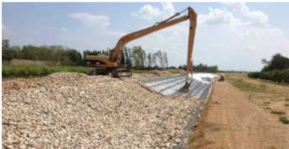
Figure 2.35. Typical photo of non-woven geotextile below revet mattress during construction
