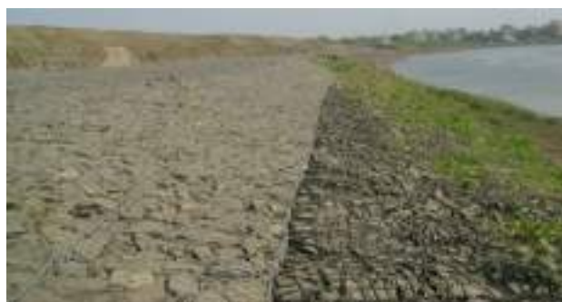
Figure 2.15. Use of gabions for river bank protection
