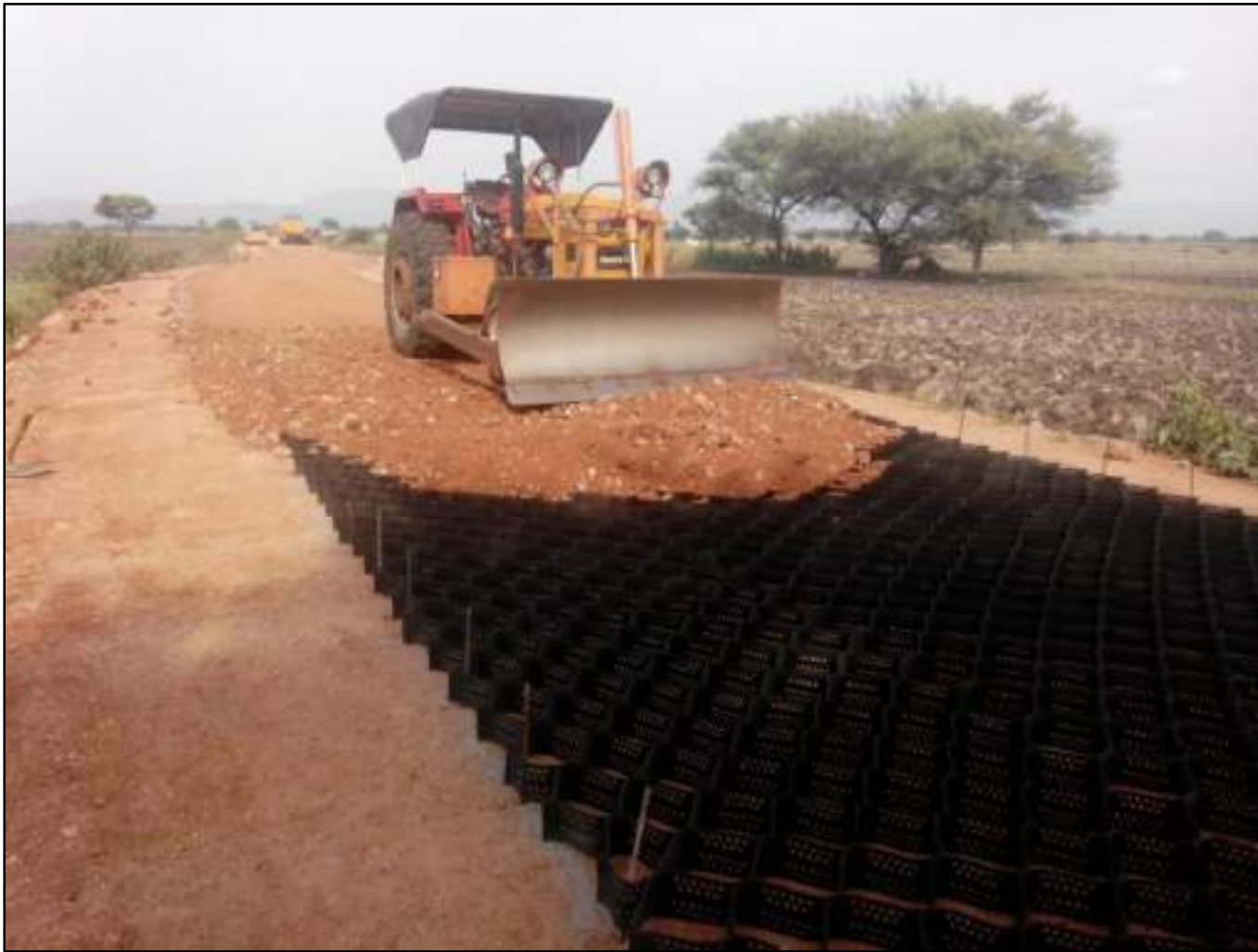
Fig. Laying of geocell and placing of infill
