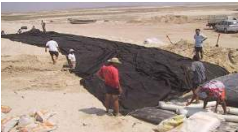
Figure 2.20. Geotube laid flat on levelled surface
