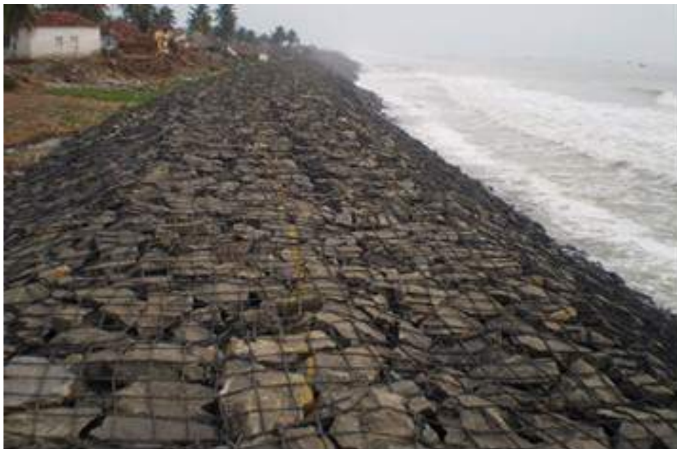
Figure 2.10. View of geotubes covered with armour protection layer of gabions
