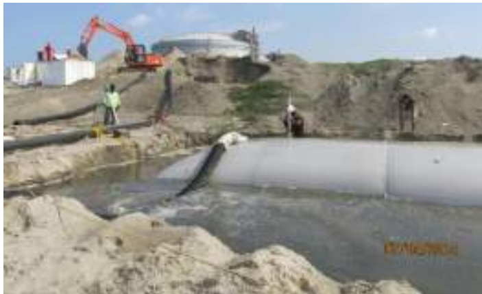
Figure 2.24. Filling of tubes
