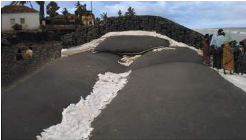
Figure 2.9. Geotubes with gabions as armour protection layer
