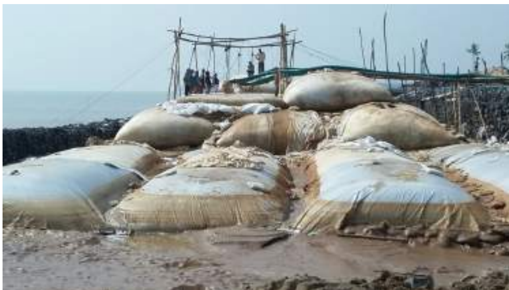
Figure 2.11. Geotubes stacked one over other
