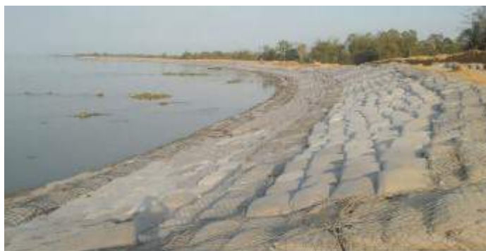
Figure 2.14. Geotextile bags for coastal protection
