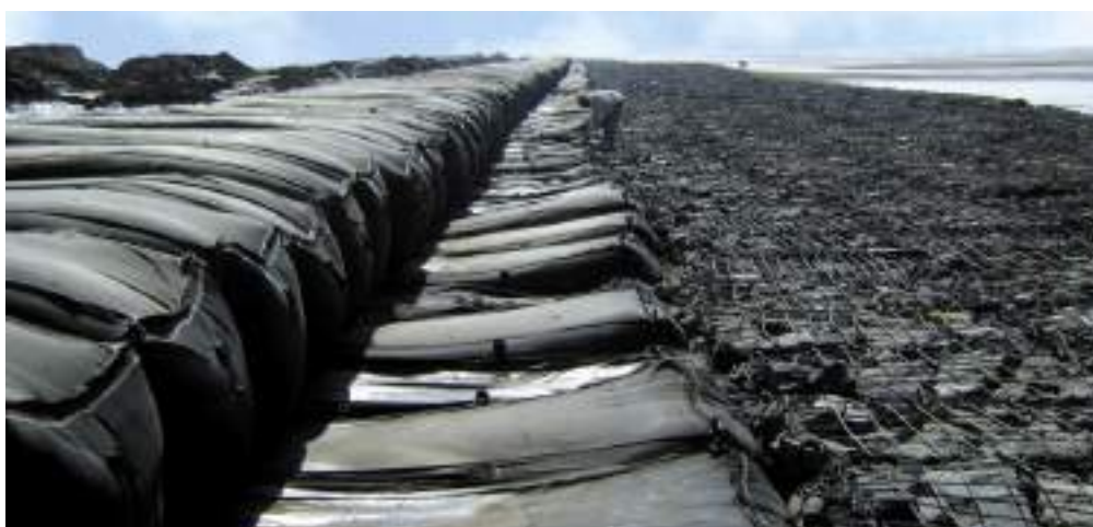
Figure 2.12. Shore reclamation using geotextile bags
