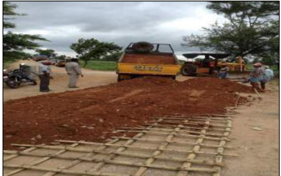
Fig. Laying of bamboo and placing of infill
