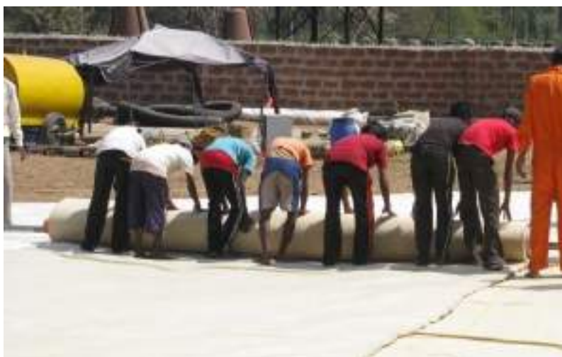
Figure 2.21. Rolling out of geotubes
