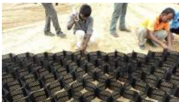
Figure 4.1 Geocell panels being laid out for road
