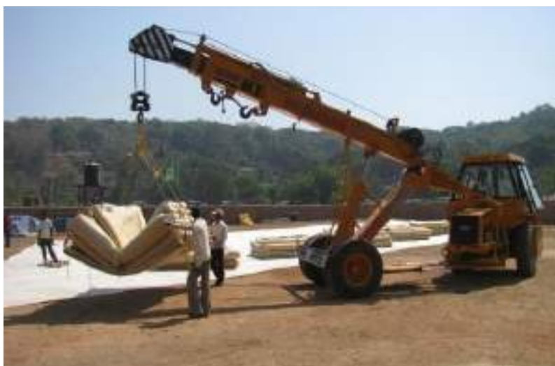
Figure 2.22. Lifting of tubes in concertina style
