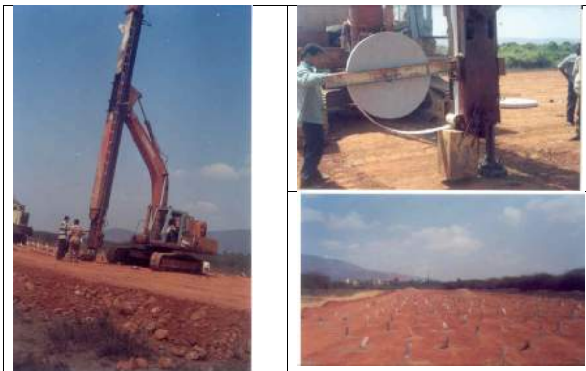
Figure 3.2. Installation of band drains
