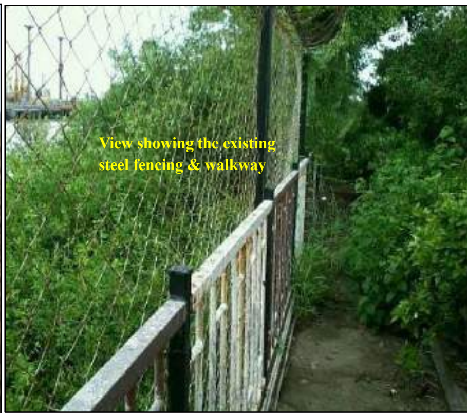
A view from chainage 840 to 940m
