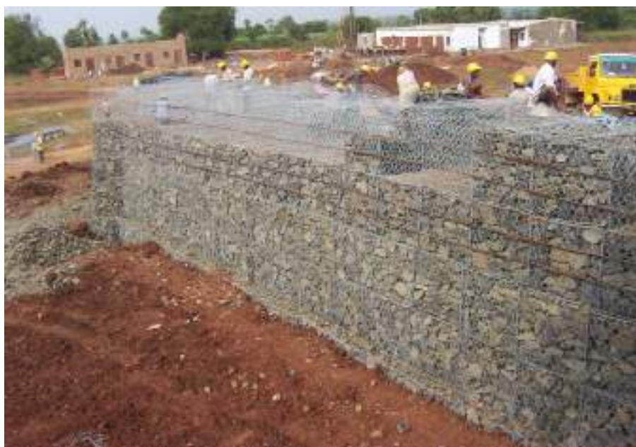
Figure 2.34. Lid closing procedure at the site
