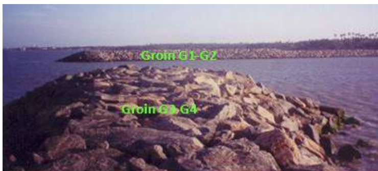
Groins at Arokiapuram
