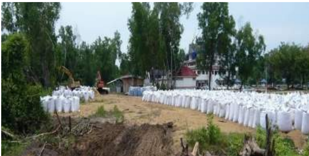
Figure 2.29. Storing of geotextile bags post filling
