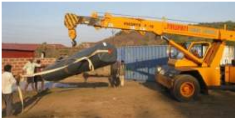
Figure 2.18. Material unloading using crane at site
