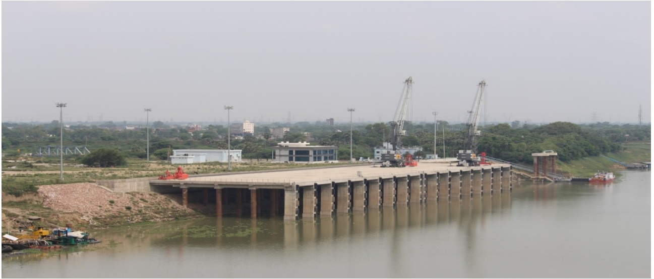
Varanasi Multi-Modal Terminal
