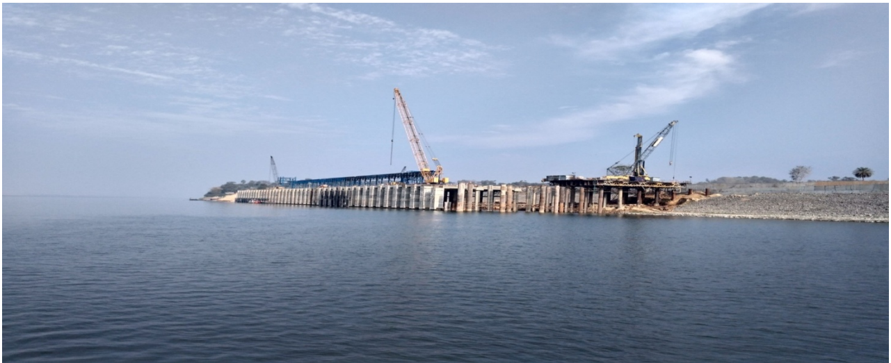
Sahibganj Multi-Modal Terminal
