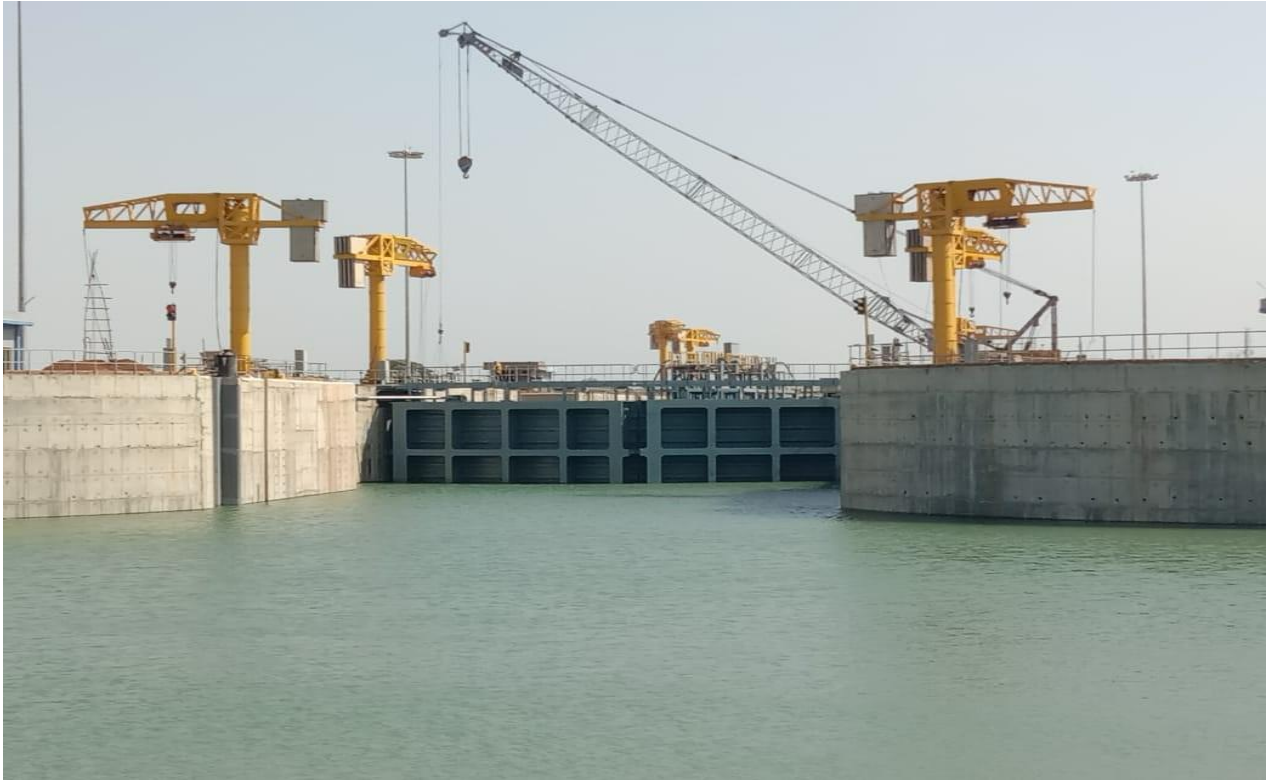
Navigational Lock at Farakka
