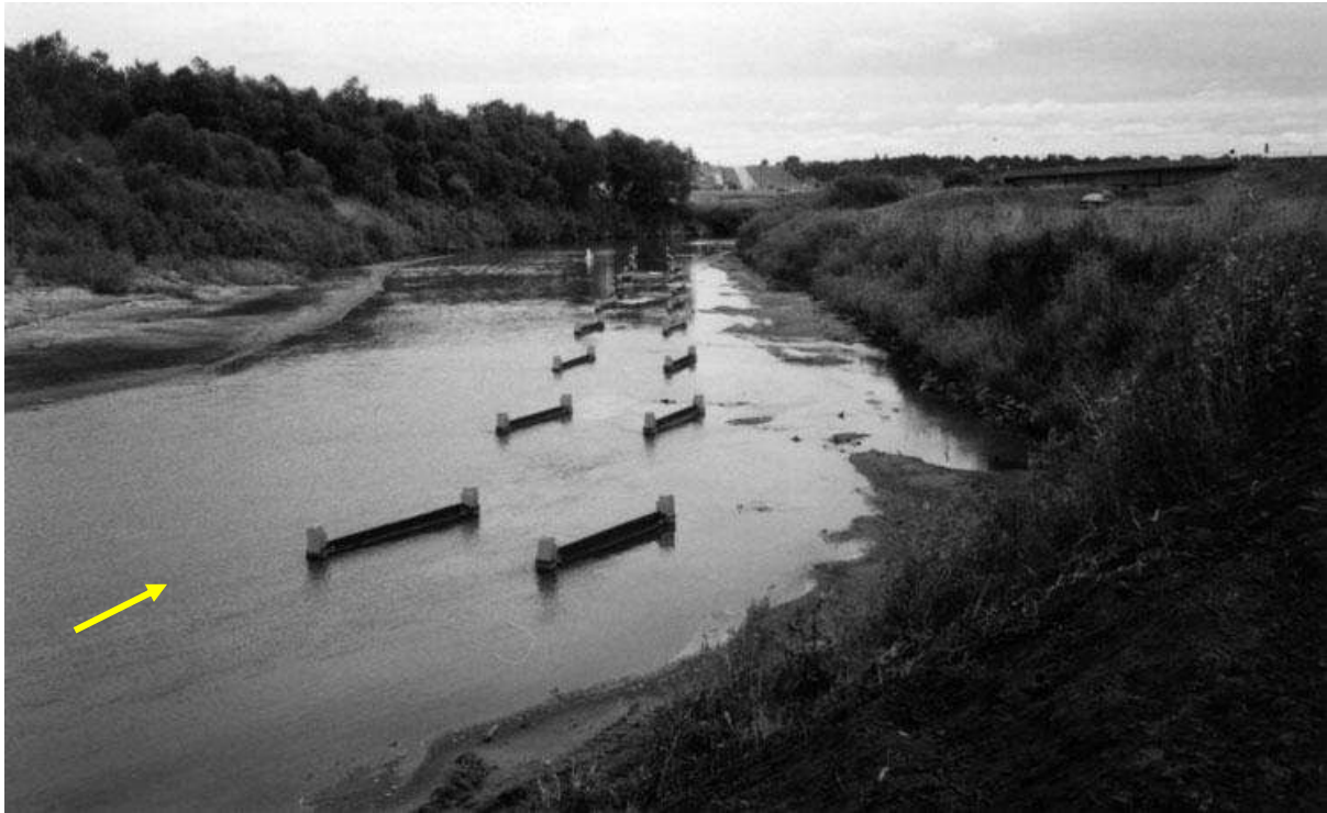
Fig. 1.3 Submerged vanes in East Nishnabotna River, Iowa, protecting stream bank against erosion (Odgaard 2009)
