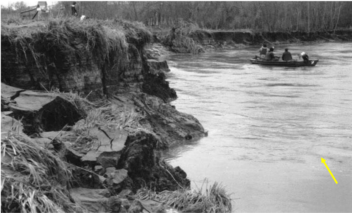
Fig. 1.1 Stream bank erosion in East Nishnabotna River, Iowa. Source: Odgaard (1987)
