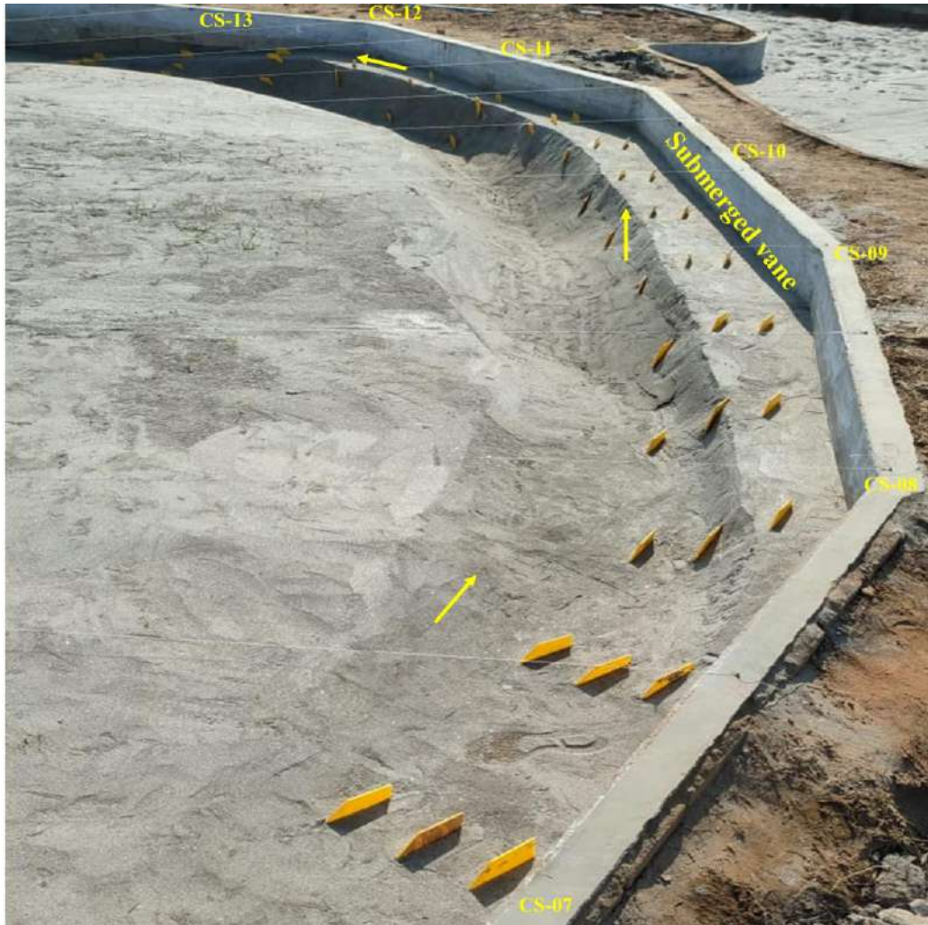
Fig. 7.5(b) Installation of vane array at right bank of the physical model
