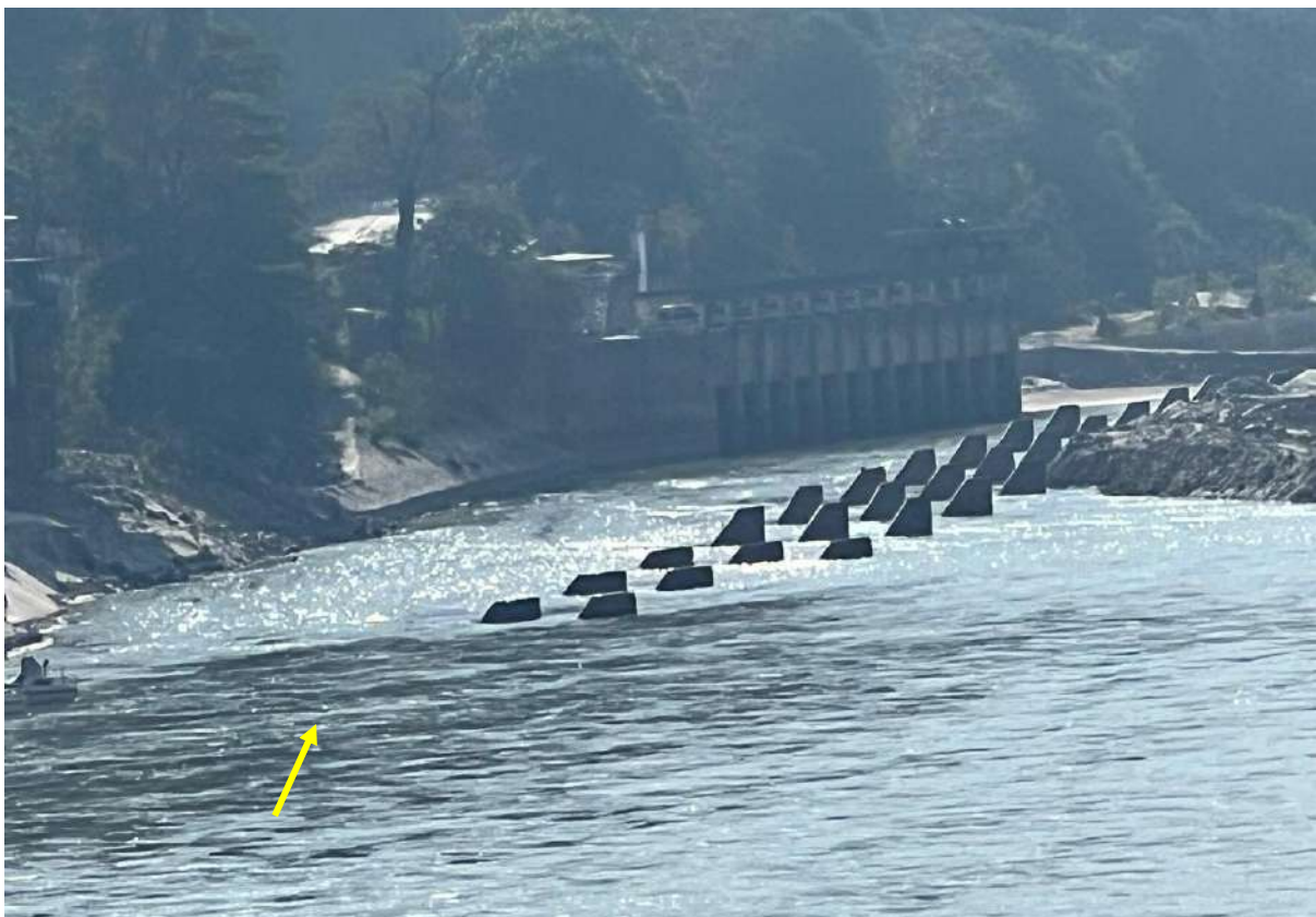
Fig. 1.4 Submerged vanes being installed at water intake on Kosi River, Nepal
